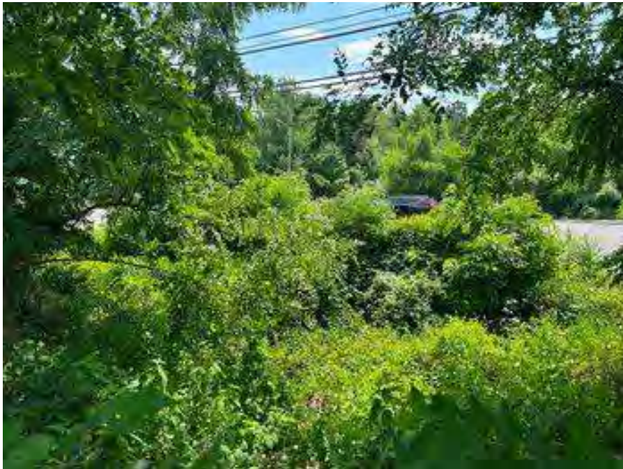
Downstream Embankment and Downstream Condition
