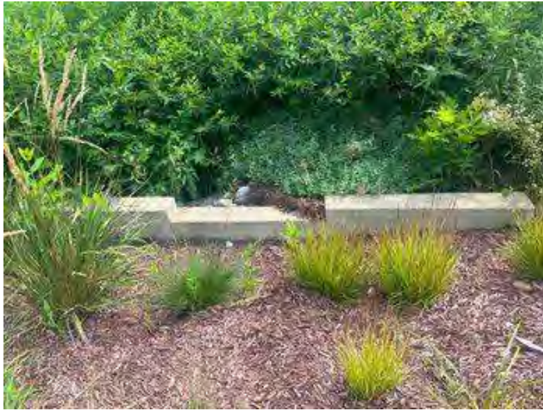
Weir wall from forebay
