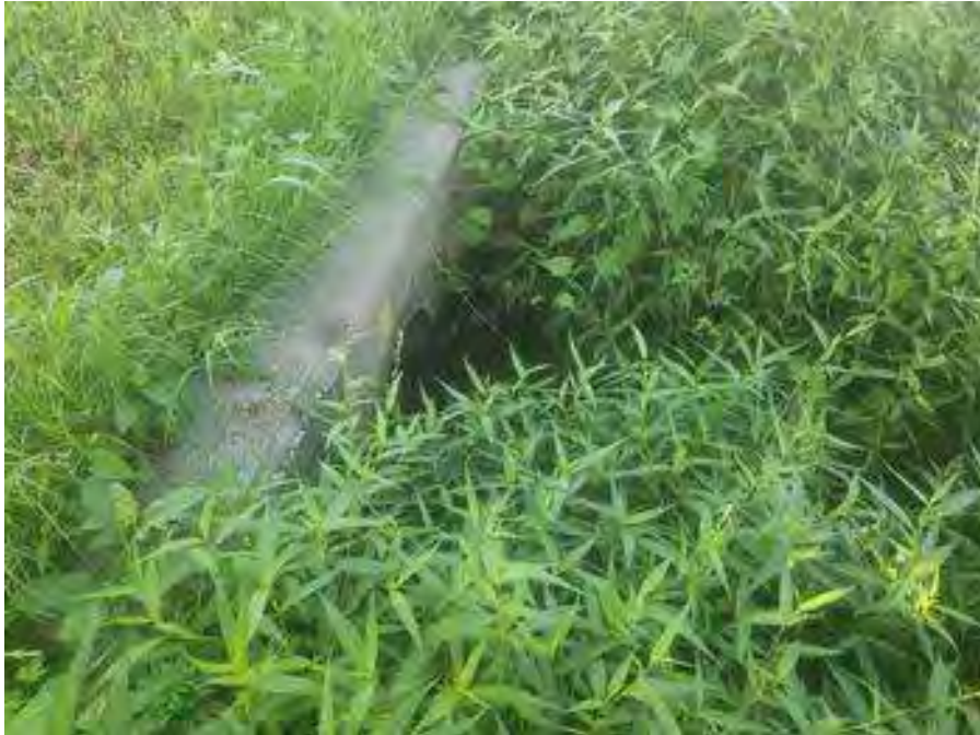
Inflow with Overgrown Vegetation
