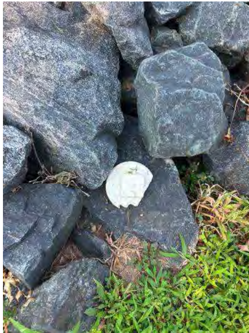
Debris in Discharge Area Close Up
