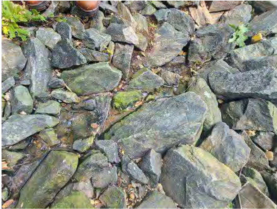
Dry weather flow Close Up in Inflow 1 Rip Rap
