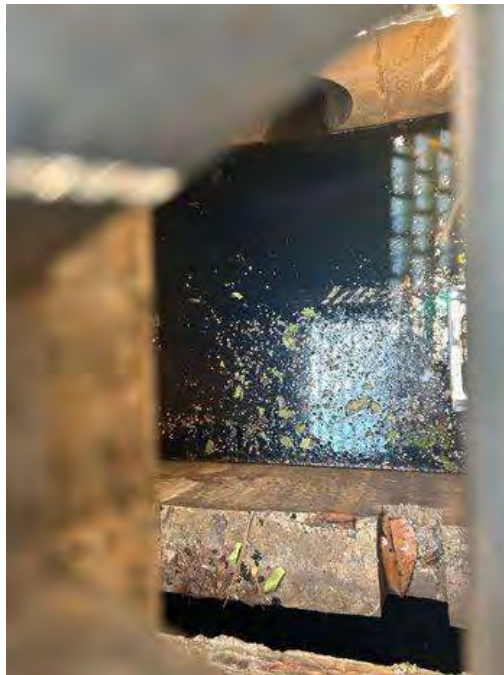
Spillway and Minor Algal Growth B
