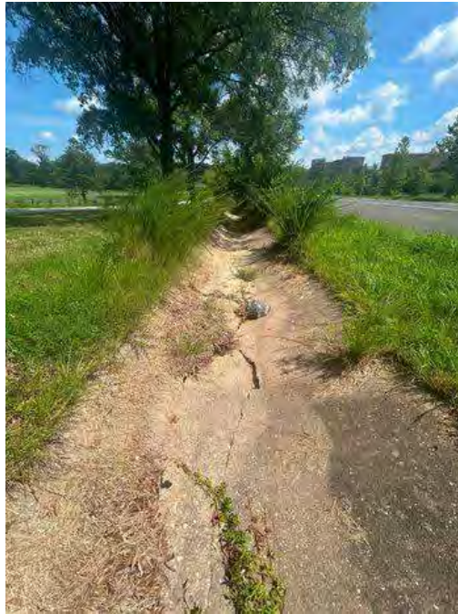
Cracked Outfall
