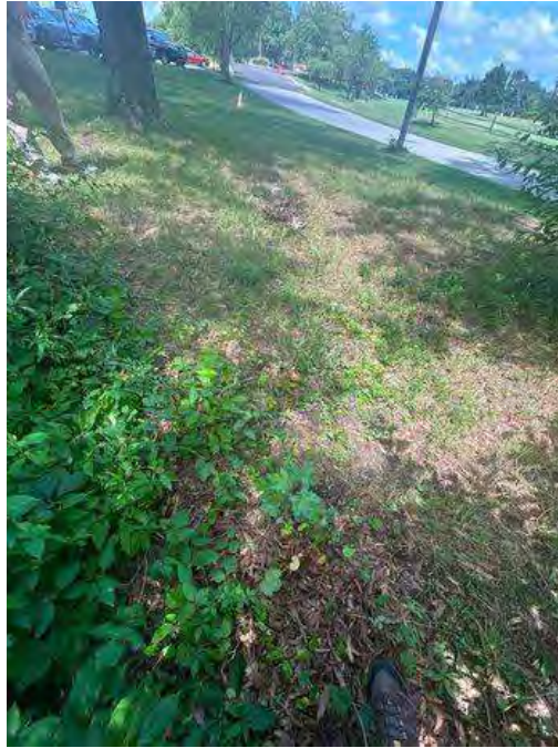
Collapsed Inflow Pipe with Discharge to Treatment Area
