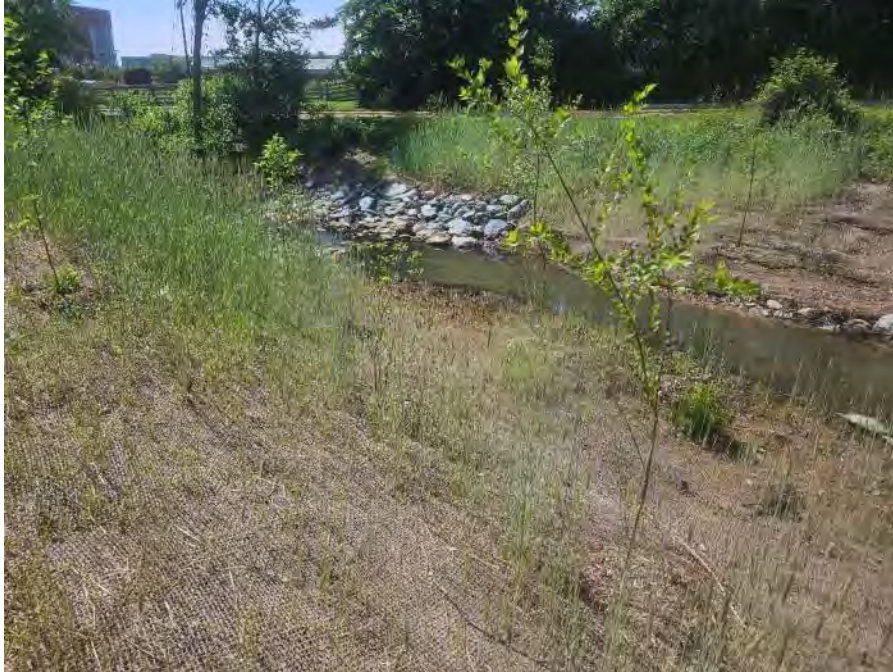
Soil Stabilization Matting and Bank
