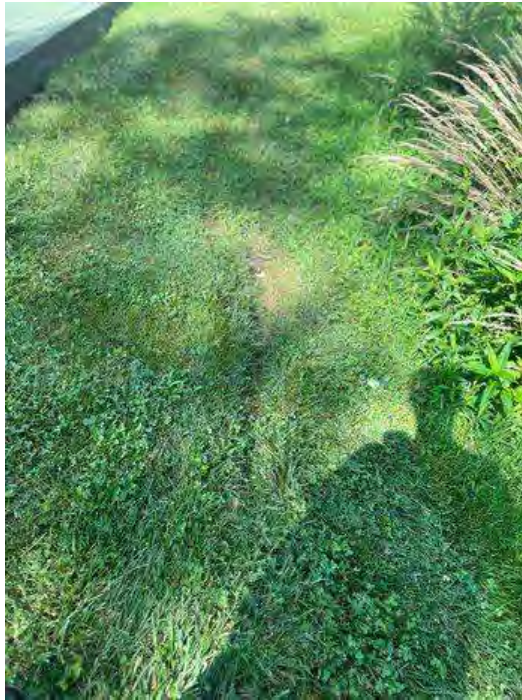
Erosion on south berm
