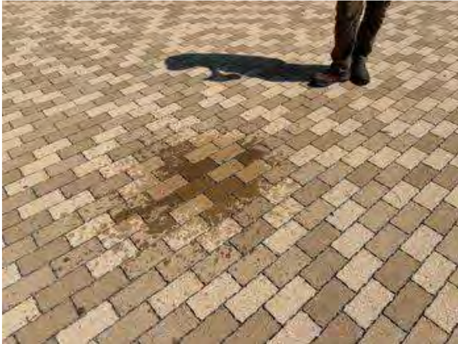
Water test flows into pervious surface
