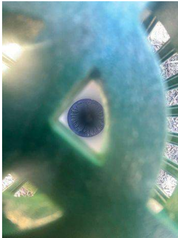
Inside of monitoring well
