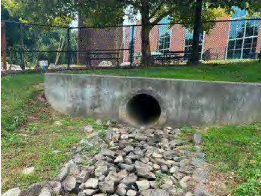
Principal Spillway Overall
