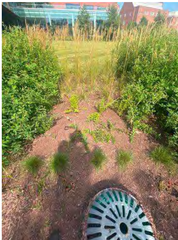
Embankment at control structure 2
