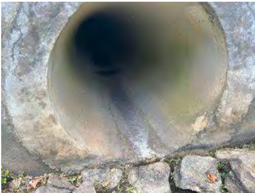
Principal Spillway Close Up
