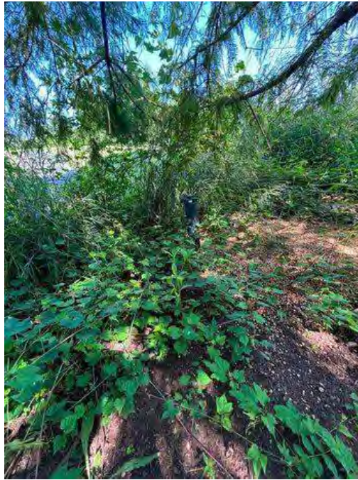
Bare Spots in Treatment Basin 3
