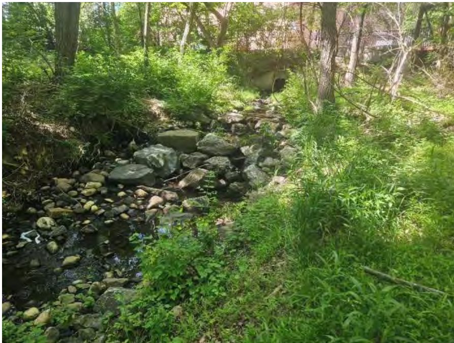
Step Pools at Outfall Channel
