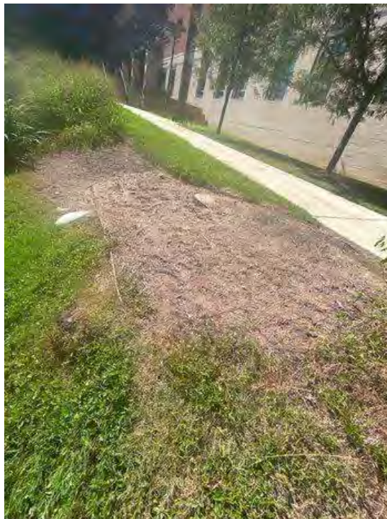
Bare area on slope
