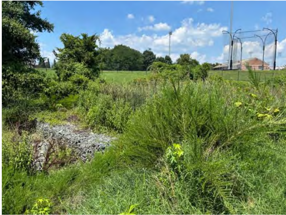
Gabion basket between east forebay and treatment basin
