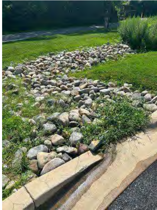
Inflow from parking lot
