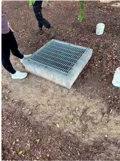
Control Structure Close Up
