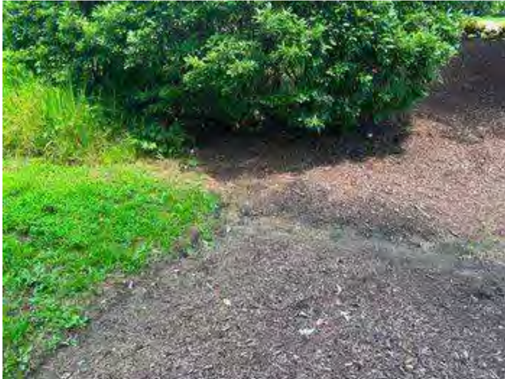
Minor sediment erosion at inflow
