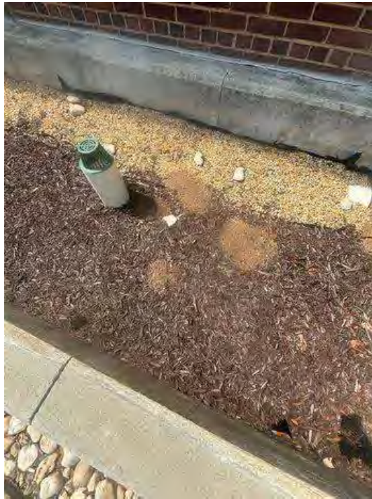
Monitoring well with emergency spillway and dirt piles in treatment basin
