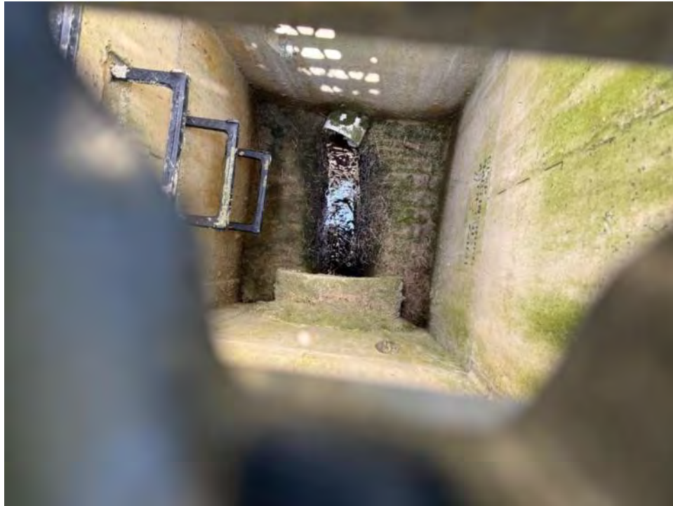
Principal spillway and underdrain inside control structure
