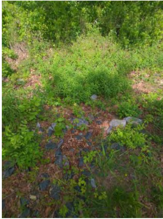
Debris in Channel
