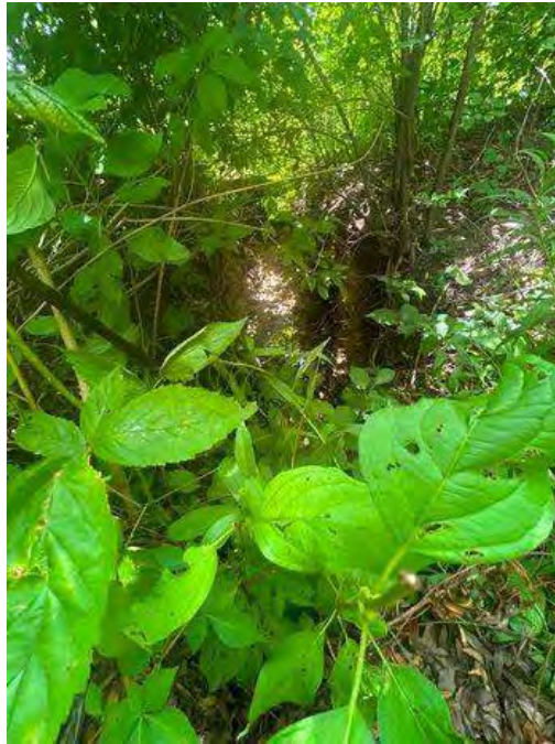
Eroded Channel Near Outfall 1
