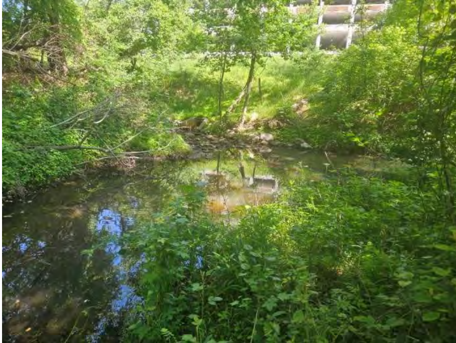
Outfall from Parking Garage
