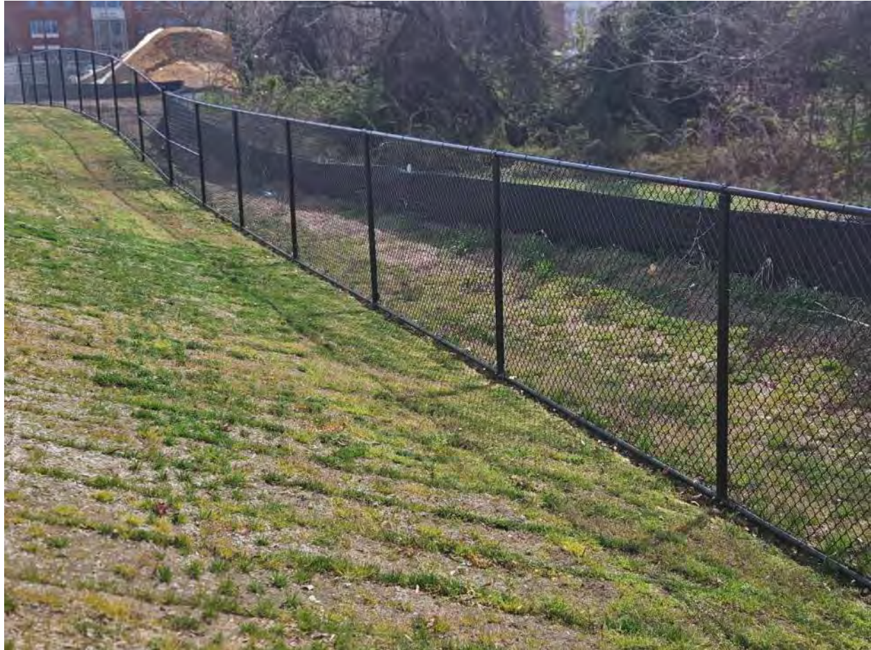
Upstream Portion of Swale
