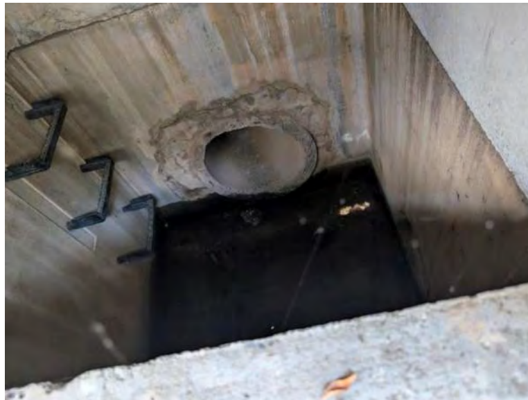
Control structure interior
