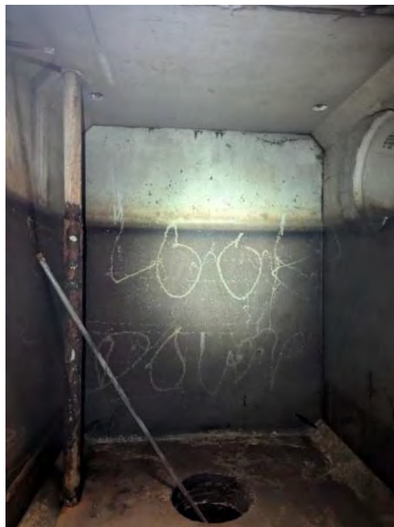
Connection to irrigation
