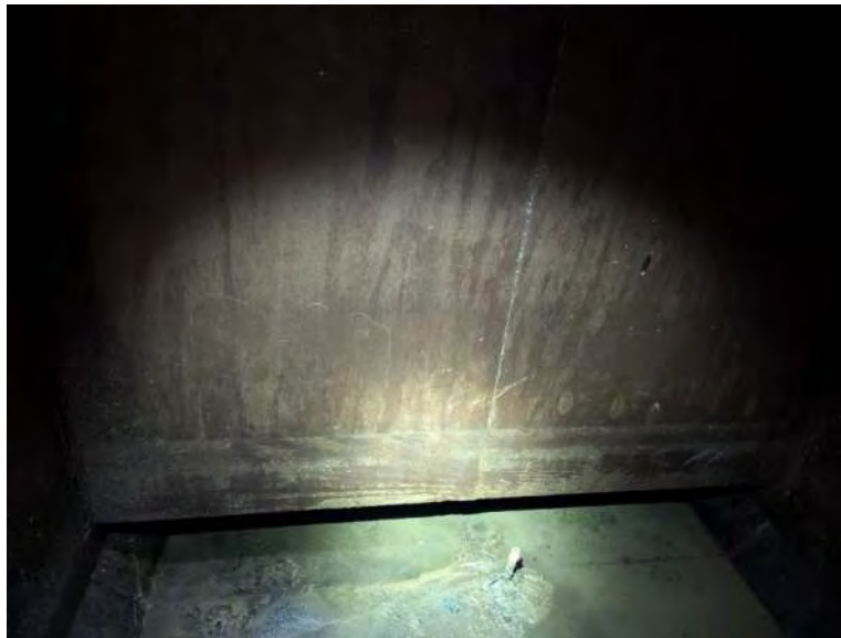
Spillway from inflow chamber
