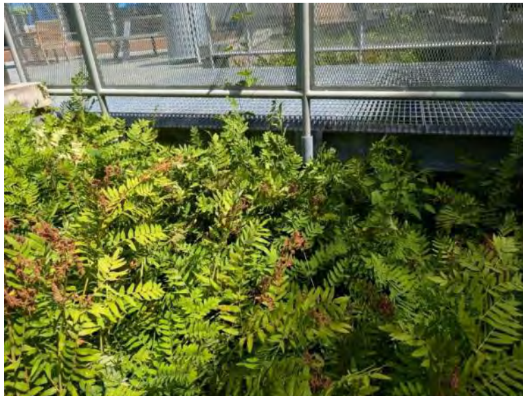
Upstream Overgrown Vegetation/Bridge over bioretention
