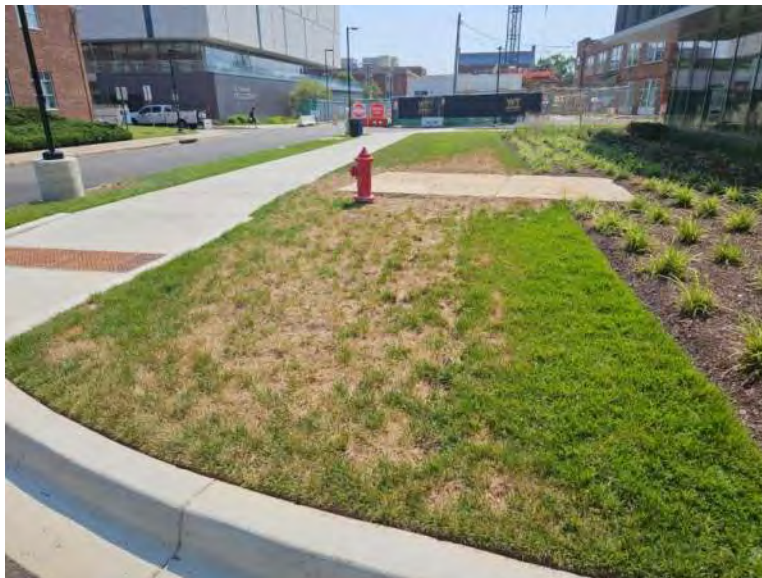
Erosion Affecting Grassy Area
