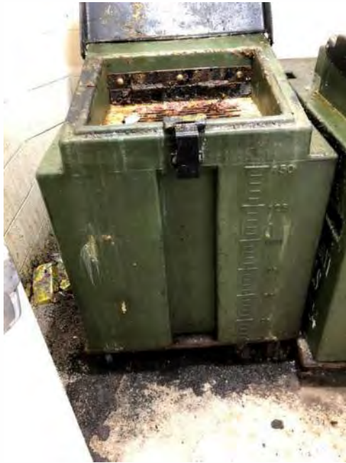
Spillage and absorbent around tank, no signage.
