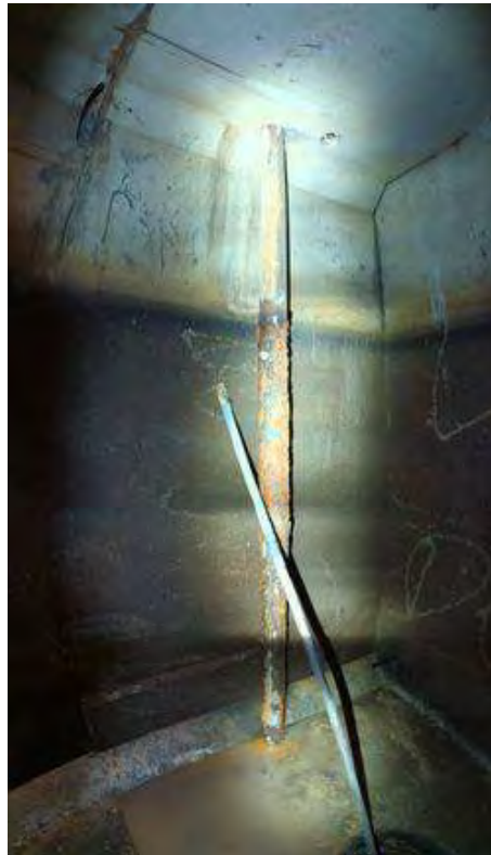
Connection pipe to irrigation
