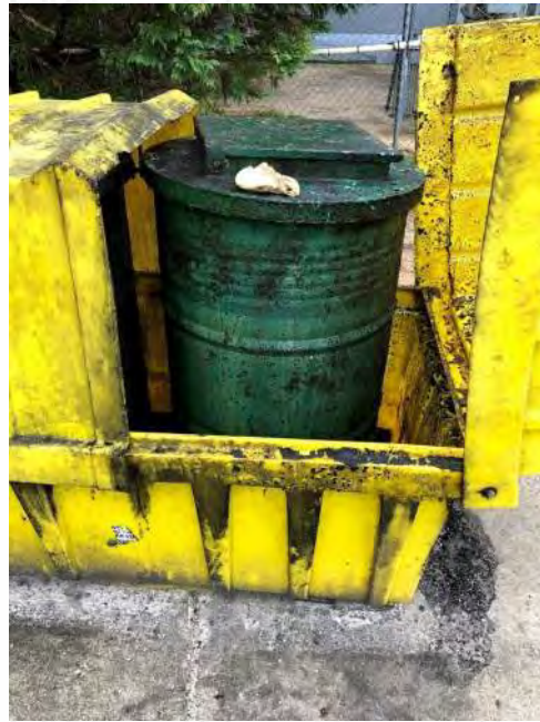
Containment not closed, spillage, no spill kit, no signage.
