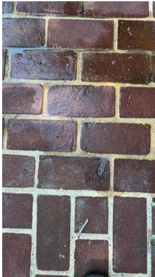
Photo Showing Permeable Pavers Have Been Grouted
