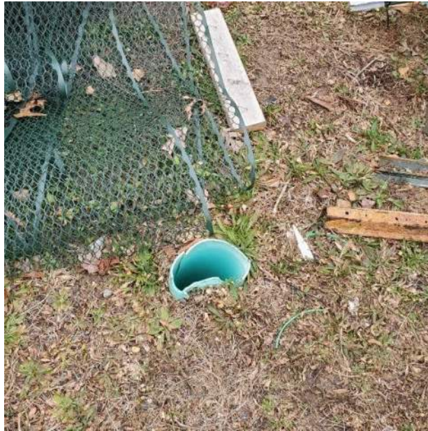
Cleanout – Replace top
