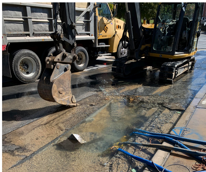
Water main leak repair
