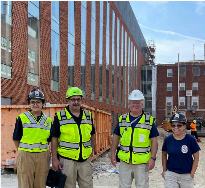
OFM Fire FP Engineers at Chemistry Wing 1
