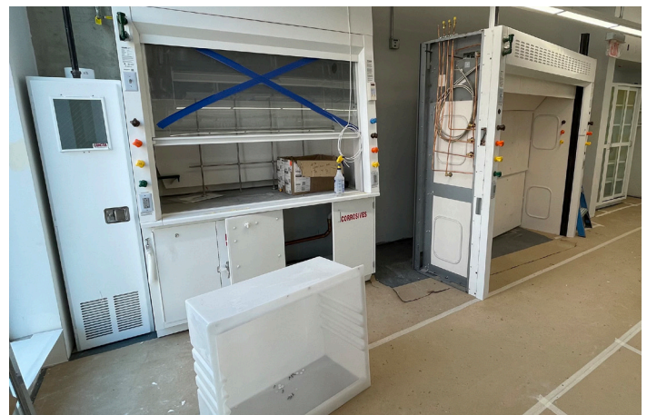
Chemistry Wing 1 Laboratory Construction
