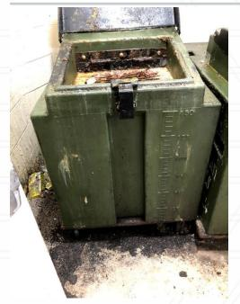
Spillage and absorbent around tank, no signage.
