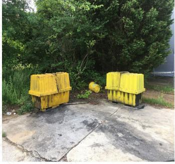
Containments are stained and have grease on the exterior, they are located in close proximity to the grassy areas, no spill kits.
