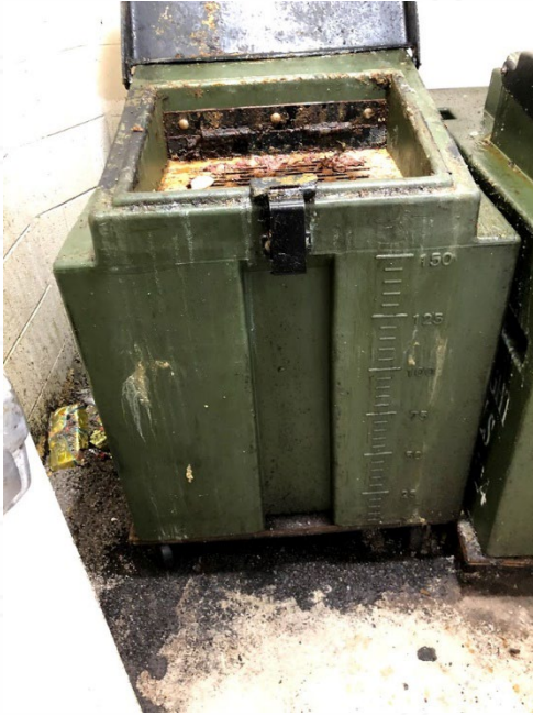
Spillage and absorbent around tank, no signage.
