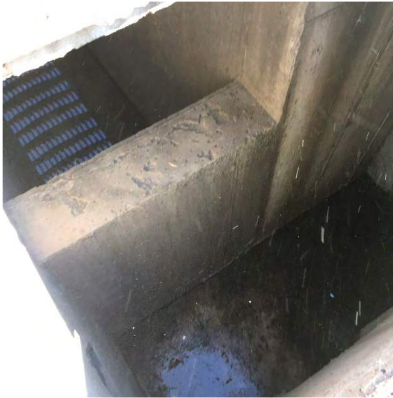
Overflow Weir & Chamber
