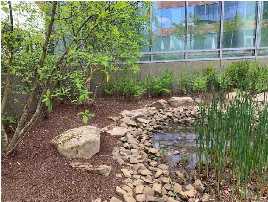
Excessive Ponding
