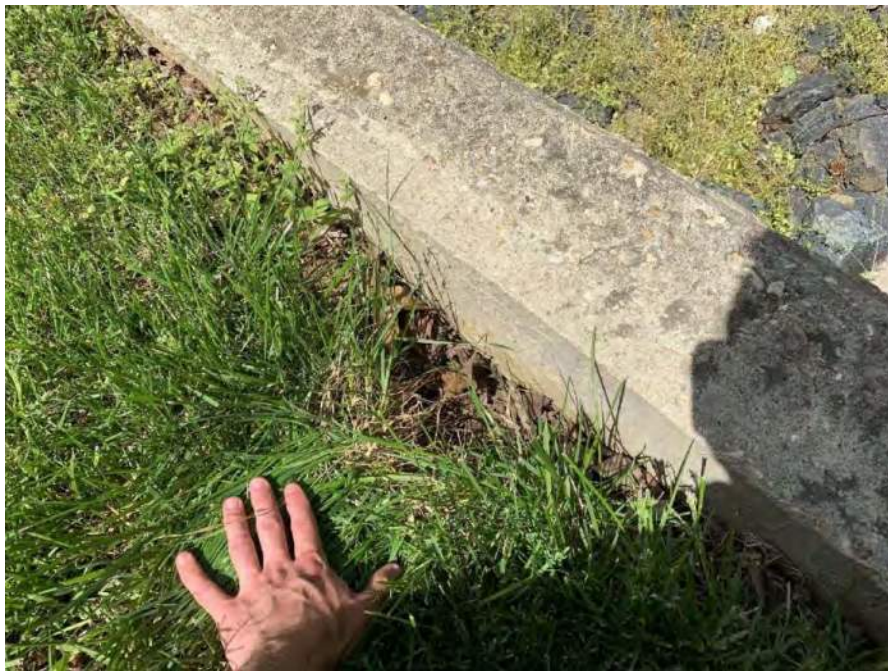
Erosion Outfall Endwall
