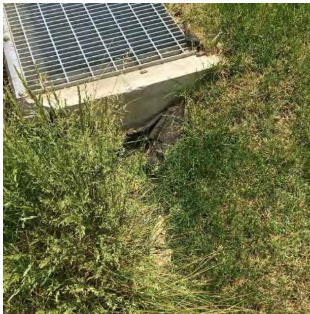
Exposed Matting Control Structure
