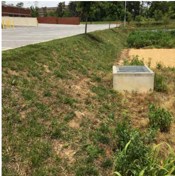
Embankment Erosion A
