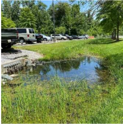
Figure 4. Ponding at Swale A south inflow
