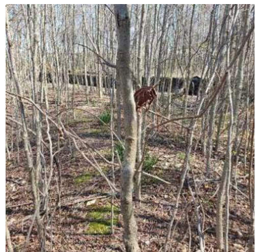
Figure 3. Tree Growth on Embankment
