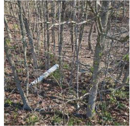
Figure 4. Overgrown vegetation at outfall
