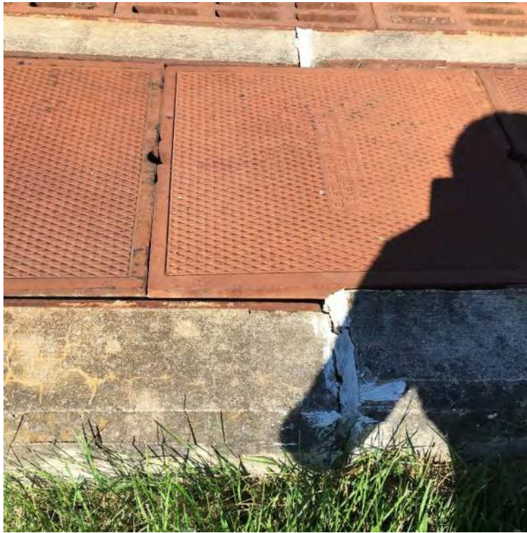
Displaced Iron Slab
