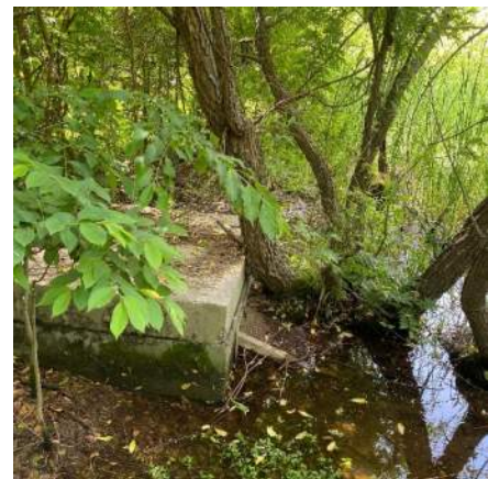
Figure 3. Tree growth at control structure
