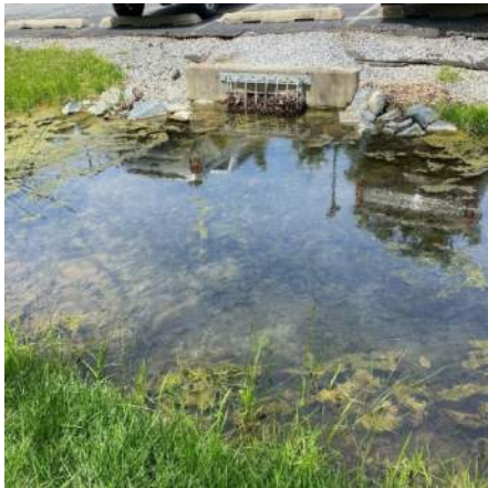
Figure 6. Ponding at Swale A south inflow and parking lot
